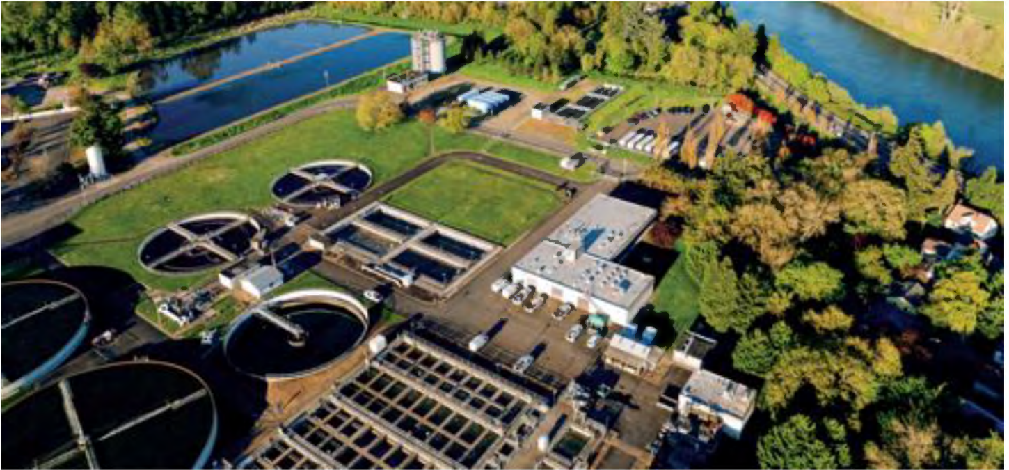
The Willamette River flows past the Corvallis Wastewater Reclamation Plant. Credit: Evan Benally Atwood
